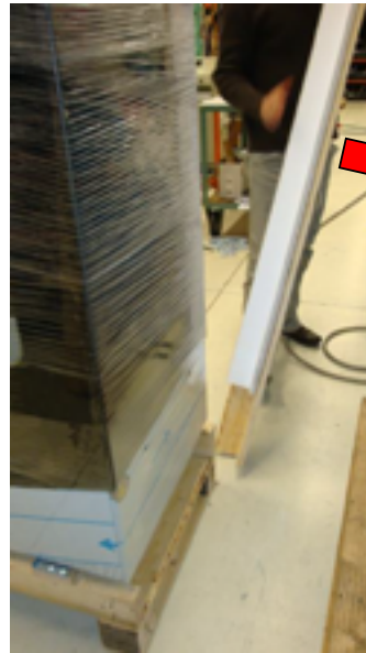
Remove vertical beams and protection on backside
